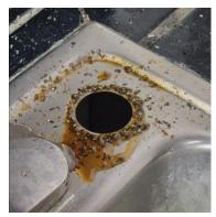
Clean up the hole, remove the excess oil, then install the side spray.
